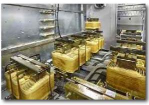
designed to minimize power factor and waveform distortion. Each load inductor coil is air cooled and thermally protected with thermal switches embedded within each coil winding. Inductors are
