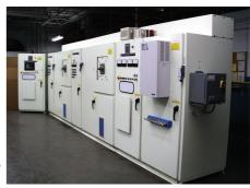
Model 506 6-pulse system for automotive e-coat.
