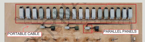
Custom Built Panels
