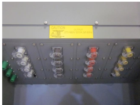
Fig 2- Inlet – Backup Generator Single Pin Connections
