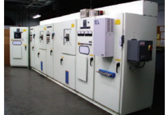
Model 506 6-pulse system for automotive e-coat.
